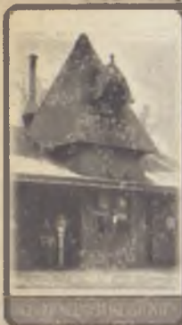
THE TOWER OF KILMORE
